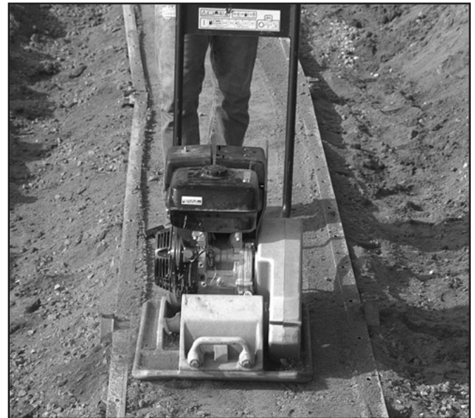
4. Compact leveling pad granular material.
