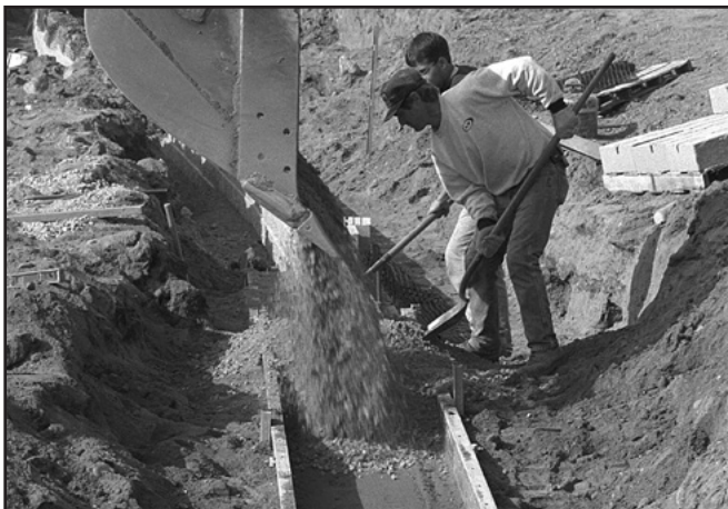
3. Fill forms with granular base material.
