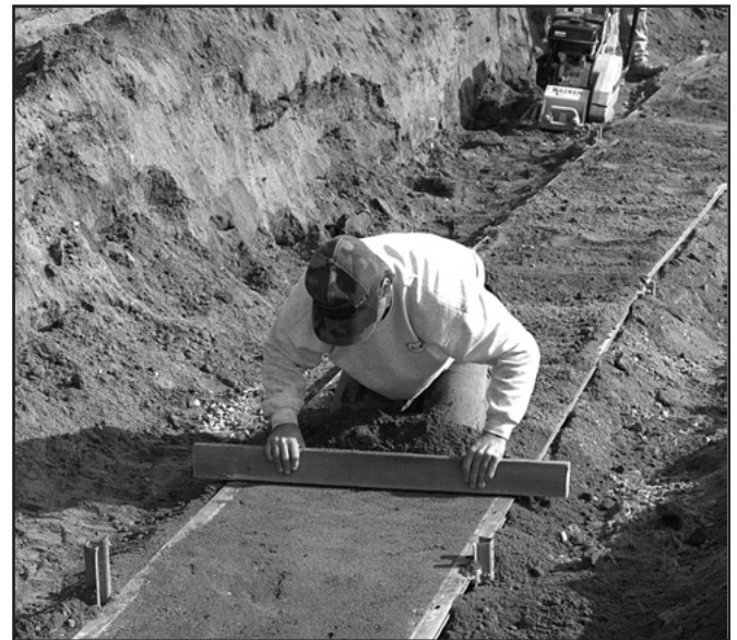
5. Screed sand for final leveling of pad.
