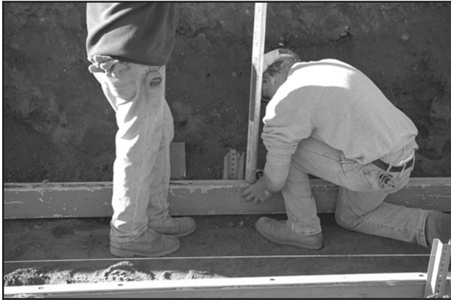
1. Set and level metal screed forms.
